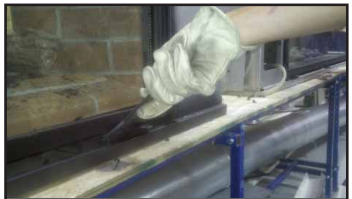
Figure 14.8. Inserting Glass Clip Tool
